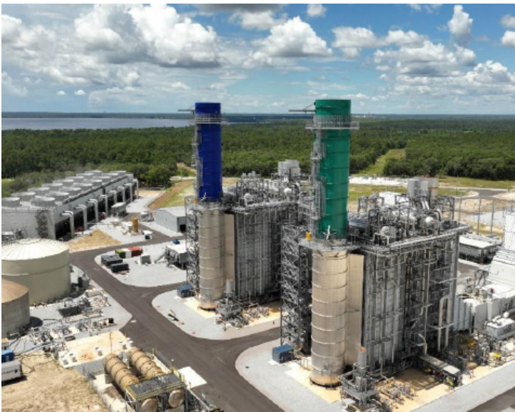
The new and improved Seminole Combined Cycle Facility, located in Putnam County, Florida, has a generating capacity of 1,134 megawatts and is one of the most efficient plants in the country, replacing one of Seminole's two coal units.
